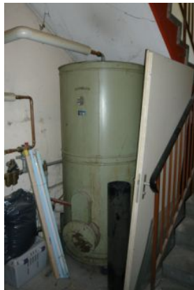
Warmwasserboiler veraltet
